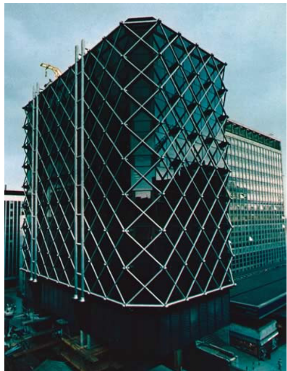
Figuur 52 Bush Lane House, London, bron [83]
