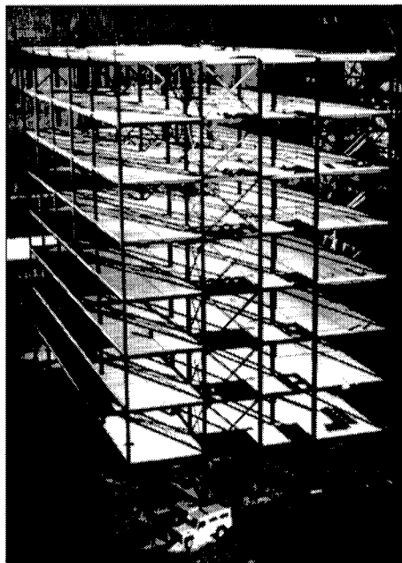
Figure 1.3 Cardington test building prior to the concreting of the floors
